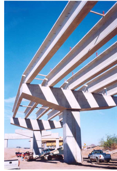
Fig. 2-4. High occupancy vehicle (HOV) lanes during construction (ADOT, 2001)
